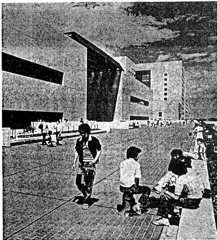
The Cooperative Restaurant and Store named "The Hilltop 78" (left), a School Library (center), and the Pedestrian Deck (foreground) are always flooded with Chuo students.
